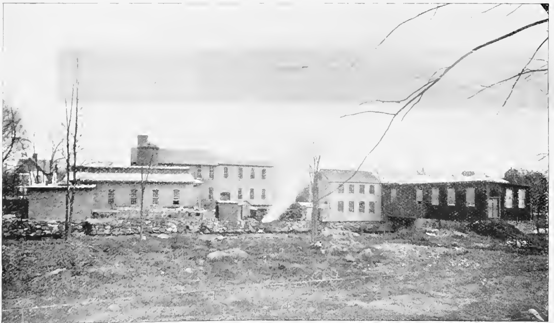
HIGHLAND MILLS—Rear View.
